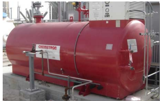
Carbon dioxide systems can be lethal when implemented improperly, which has led to strict NFPA regulations about CO 2 system application
